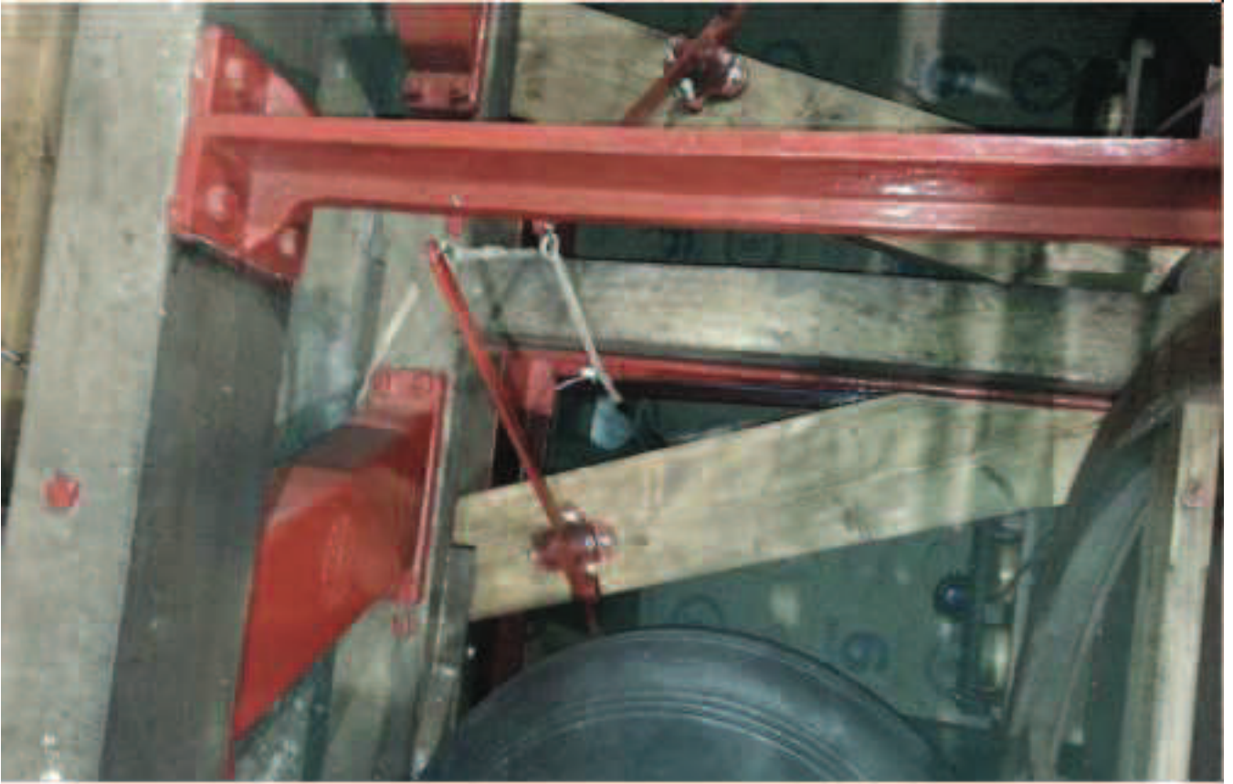
During the recent Almondsbury Bells Restoration Project (ABRP) the Ellacombe chimes were restored
